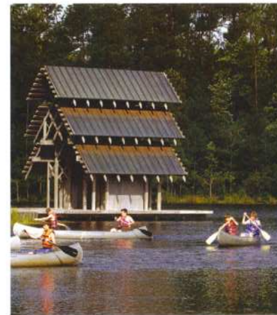
Pine Eagle Chapel, Camp Tiak Scout Camp, near Wiggins, Mississippi; Fay Jones + Maurice Jennings Architects
